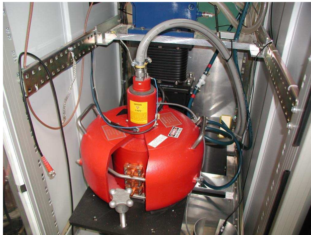
Fig. 1: Klystron VKL7811St at ELBE (1.3 GHz, 10 kW).
