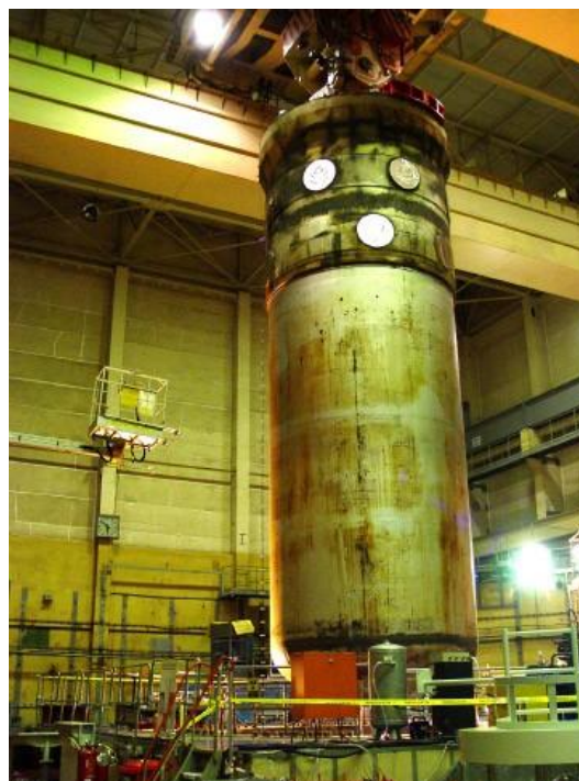
Fig. 1: RPV of the decommissioned Greifswald NPP. [1]
