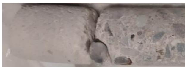
Figure 1. Measured and calculated activities of ^{60}\text{Co} , ^{152}\text{Eu} , and ^{154}\text{Eu} of a drill core from the floor below the RPV consisting of an 11 cm screed-layer on top of normal-density concrete. Bottom: Photograph of the analyzed drill core.
