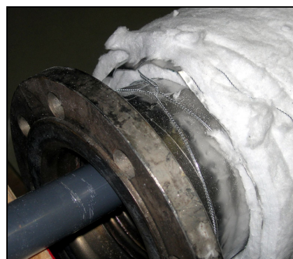
Fig. 2.12 Insulation of a hose with Superwool blanket
