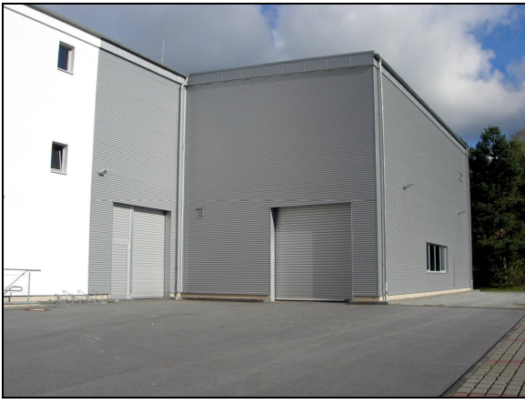
Fig. 2.2 New wing of the TOPFLOW building
