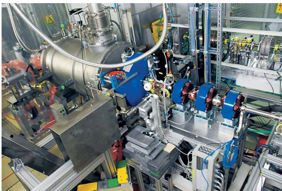
Fig. 1: SRF photoinjector in the ELBE accelerator hall. Left side: vacuum vessel with the helium transfer line on top. Right side: electron beamline with the emittance compensation solenoid, the laser input port, the first screen station, and three quadrupole magnets.
