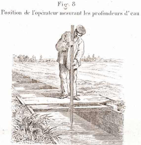
Figure 2.6: Original illustration of the measurements of Darcy & Bazin (1865)
